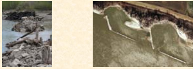
Fig 1. Notched wing dikes on the Missouri river (Corps of Engineers mitigation sites)
