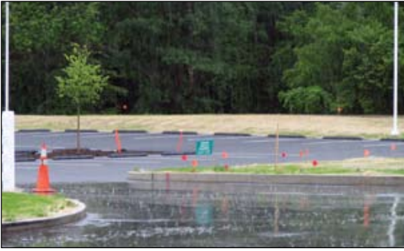
Porous Pavement Example 1: Porous pavement (background) parking lot, adjacent to conventional street during rain storm at Ryerson Woods Welcome Center. Porous pavement allows infiltration and reduces runoff (Lake County, Illinois).
